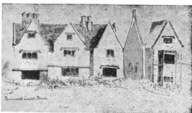
PAINSWICK COURT HOUSE (MANY GABLED HOUSE).
