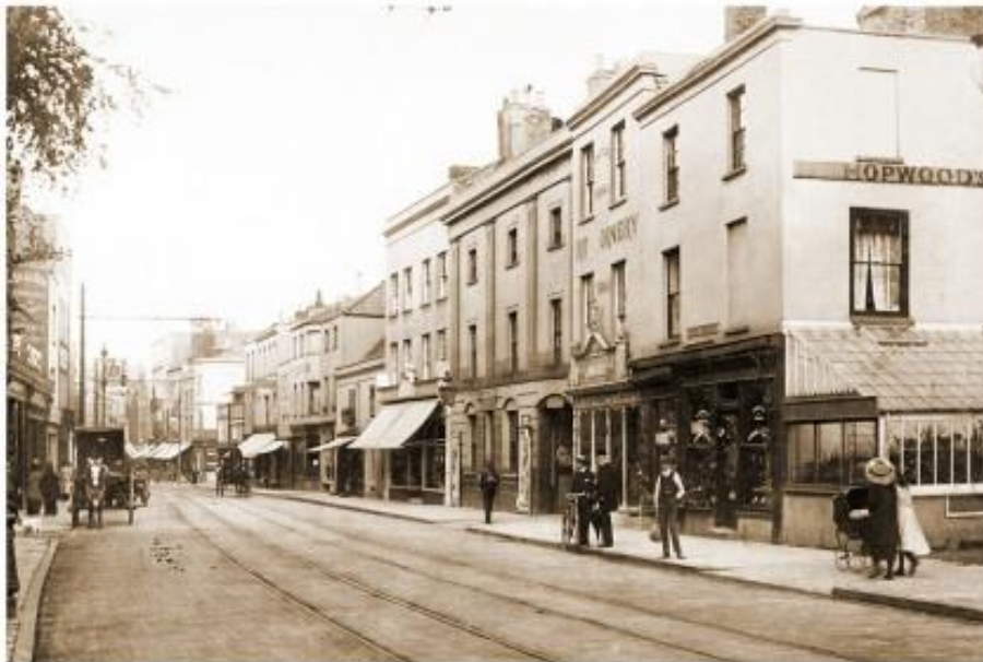
The Restoration Inn, (top, arrowed) and (below) the upper or eastern section of the High Street. The tram lines are visible in the centre, early 20 th century.
