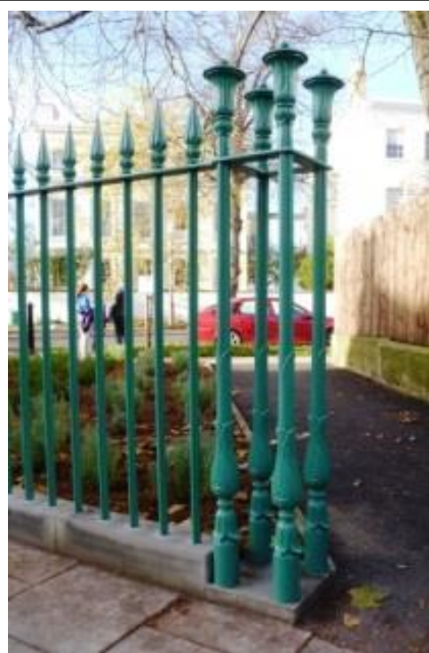
The restored ironwork of Pittville Gates shows Stokes' attention to detail and crisp design.
