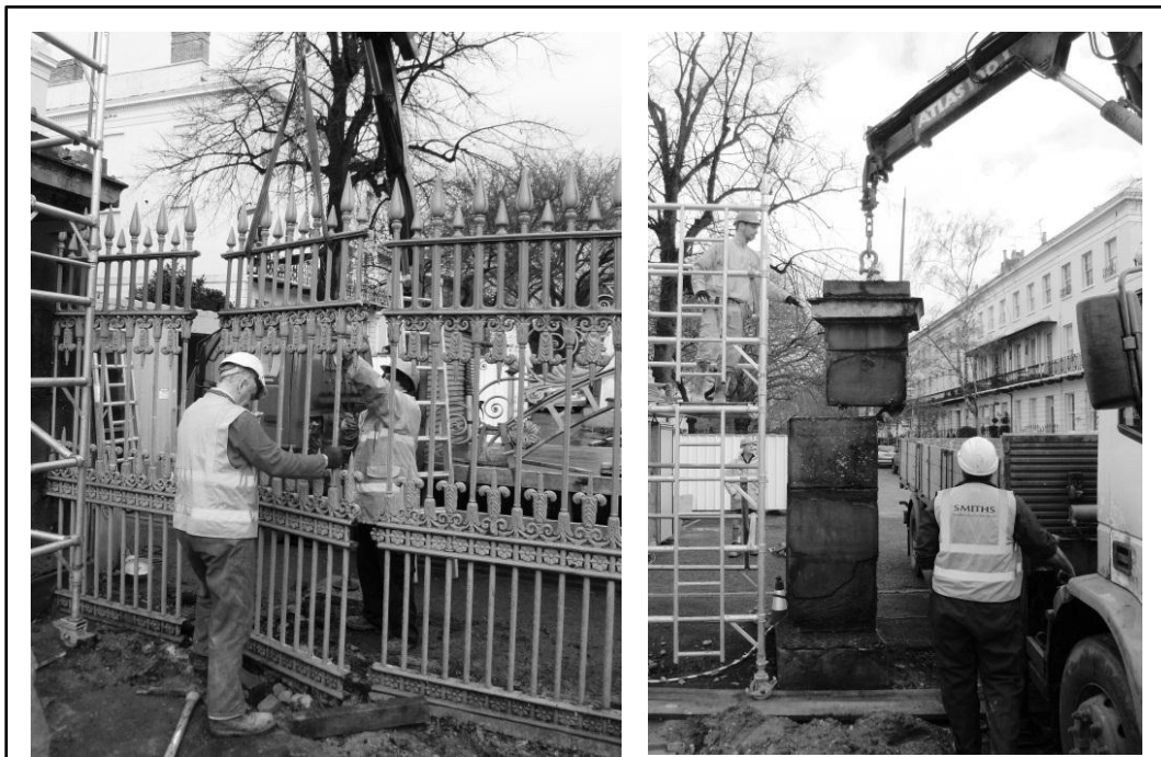
19 November 2012, workmen dismantling Pittville Gates ready for restoration
