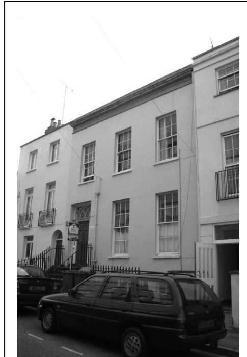
St Albans (centre) with Wellington House to the left. The space to the right that Amina describes is now infilled with a Regency-style modern building.
