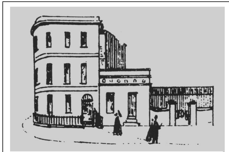
The former No. 1 Portland Square, including J.W. Berington's Ale, Porter & Cider Stores, from George Rowe's Illustrated Cheltenham Guide (1845). Now the Sudeley Arms , 25 Prestbury Road.
