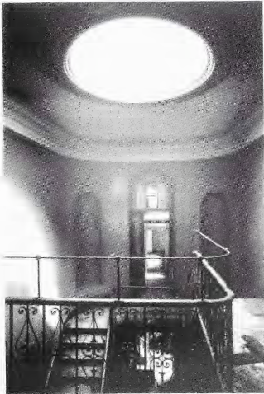
The 2nd floor landing skylight at The Priory, London Road, about 1967
