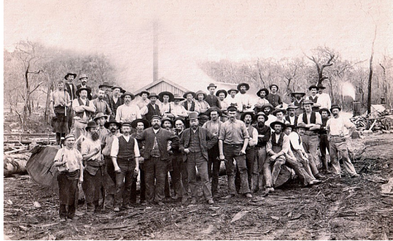
Workers at Canning Jarrah Mill, where Enoch died
