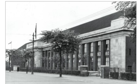
The Howitt Building, Nottingham
