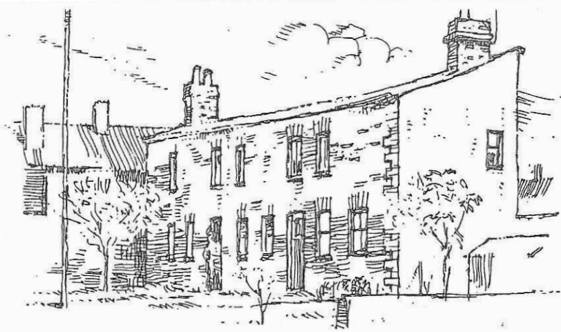
The surviving cottages in Providence Square
