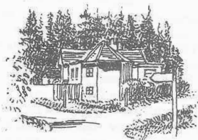
Toll House at Greenway Lane
