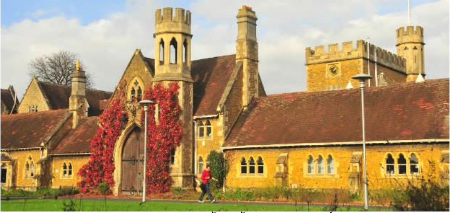
Francis Close Hall was built as a teacher training college on land donated by Jane Cook in 1848.
